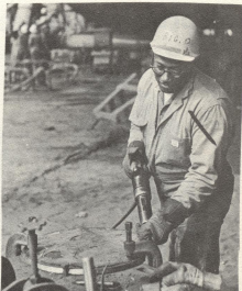
Yardworker Oliver Bolds bevels a plate which will be used to plug openings in Bena's bottom.
