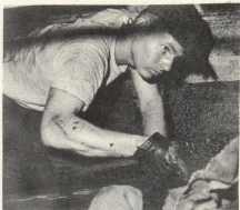
PA Louis A. Lester under a boiler using compressed air to clean air casing.
