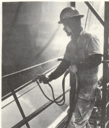
Yardworker George A. Vogel shoots on a coat of red lead primer.
