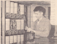
Charles Tim, ICS Checking telephone circuit to find location where receiver was left off the hook.
