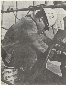
Left--Yardworker grinds clean a channel adjacent to the wooden flight deck.
