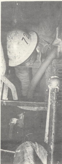
Yardworker dips suction hose into murky sump in Fireroom Number Three.
